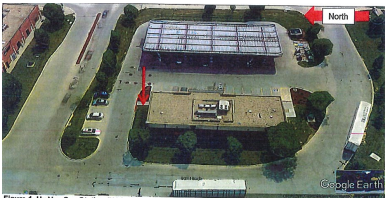
Figure 1. Hy-Vee Gas Station #10 looking east. Red arrow indicates location of air pump at time of incident. Via Google Earth.
